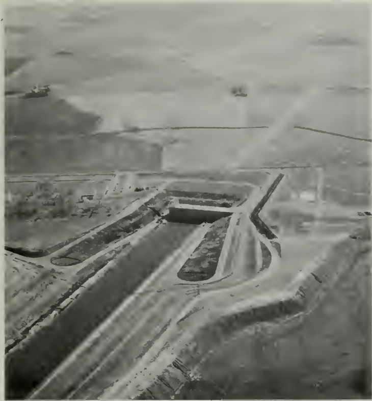
Tracy Pumping Plant
